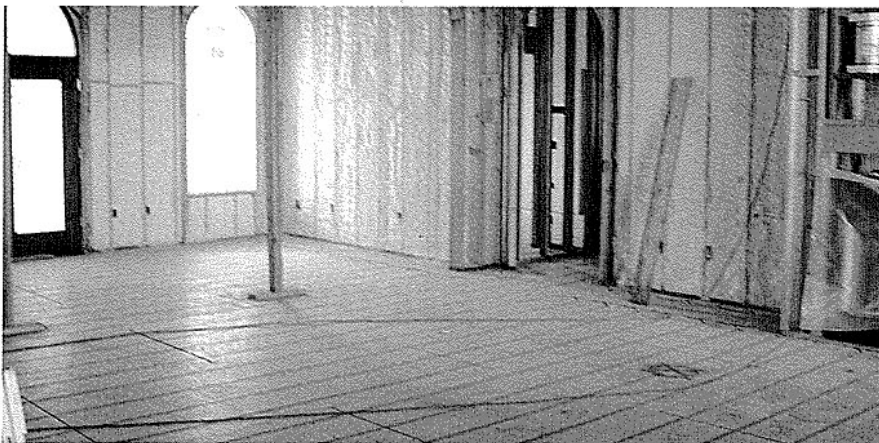
Warmboard, an integrated structural subfloor and radiant panel, distributes heated and cooled water through PEX tubing in a modular pattern of channels.
